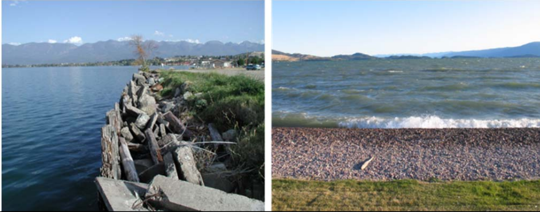
Before and after: Old sea wall (left) replaced with dynamic equilibrium beach (right) on Flathead Lake.
